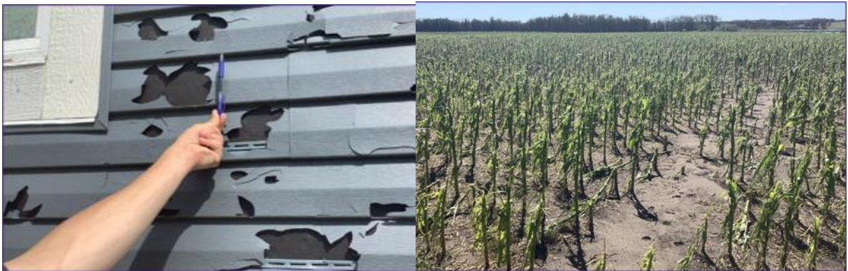
Figure 3. Severe vinyl siding damage (left) and 100% loss of corn crop (right) west of Ponoka, Alberta.
